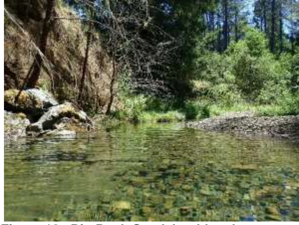
Figure 18. Big Rock Creek boulder clusters installed in the 1990s still preventing bank erosion and scouring a pool. 6/23/19.
