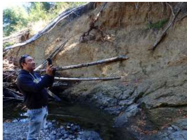
Figure 14. Tony Varnhagen and bank erosion site on his property. 9/8/19.
