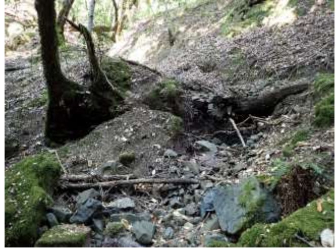
Figure 36. Tributary channel also used as skid trail, bare-banked and down-cutting.
