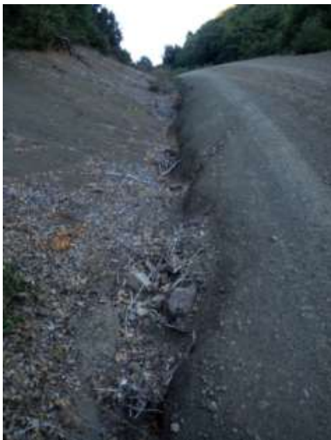
Figure 23. Gully in upper Cahto Peak Rd.
