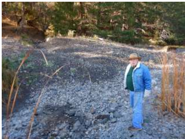
Figure 27. Landowner Bob Vassar points out major sediment deposition from gully on lower Tenmile Creek. 10/16/18.
