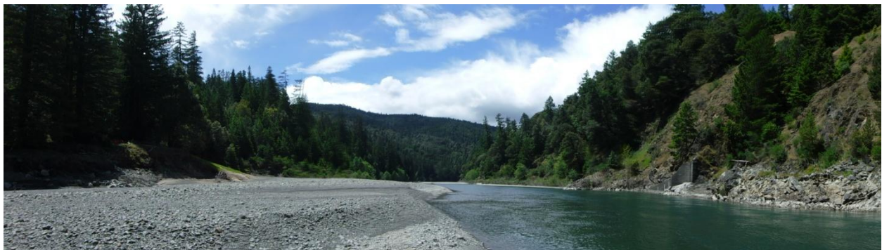
Site of old Benbow Dam with just the abutment on the right remaining. 5/13/17.
