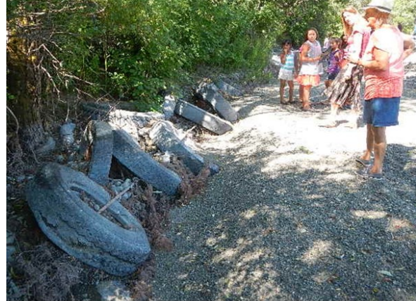
Figure 6. Cabled truck tires used to prevent Town Creek bank erosion.
