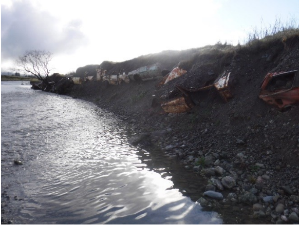
Figure 5. Car bodies used for stabilization embedded in bank.
